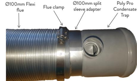
Step 2: Slide the flue clamp onto the Ø100mm flexi flue. The Ø100mm flexi flue is then slid onto the outside of the split sleeve and pushed as far down as possible.
