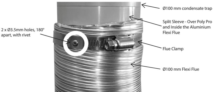
**NOTE:** The condensate drain exit tube must be in a downward position. The flue support brackets are to be used on all Poly Pro flue components.
