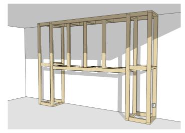
Construct the wood framing following all minimum fireplace chase opening requirements and with consideration to vent pathways. Provide a continuous base for the fireplace. Allow for mains power connection and an accessible isolation switch.
